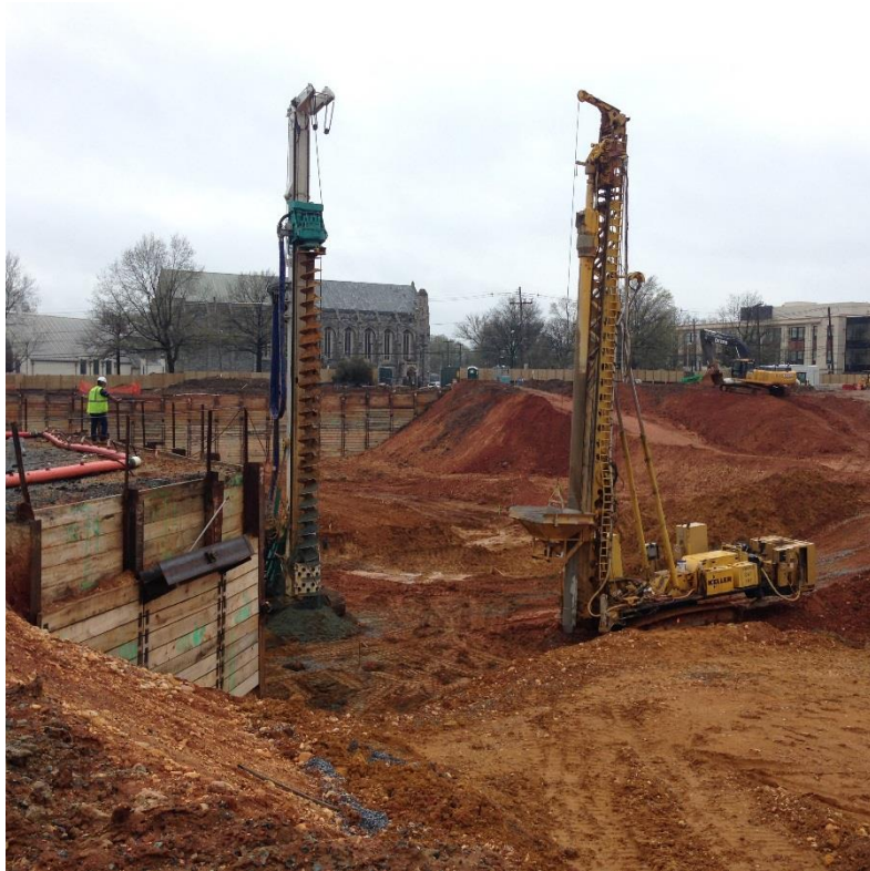
Geo-pier Installation
