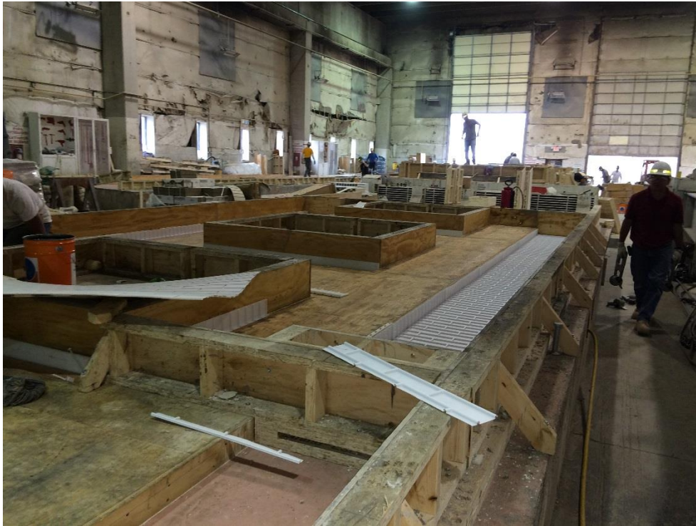
Façade prefabrication
