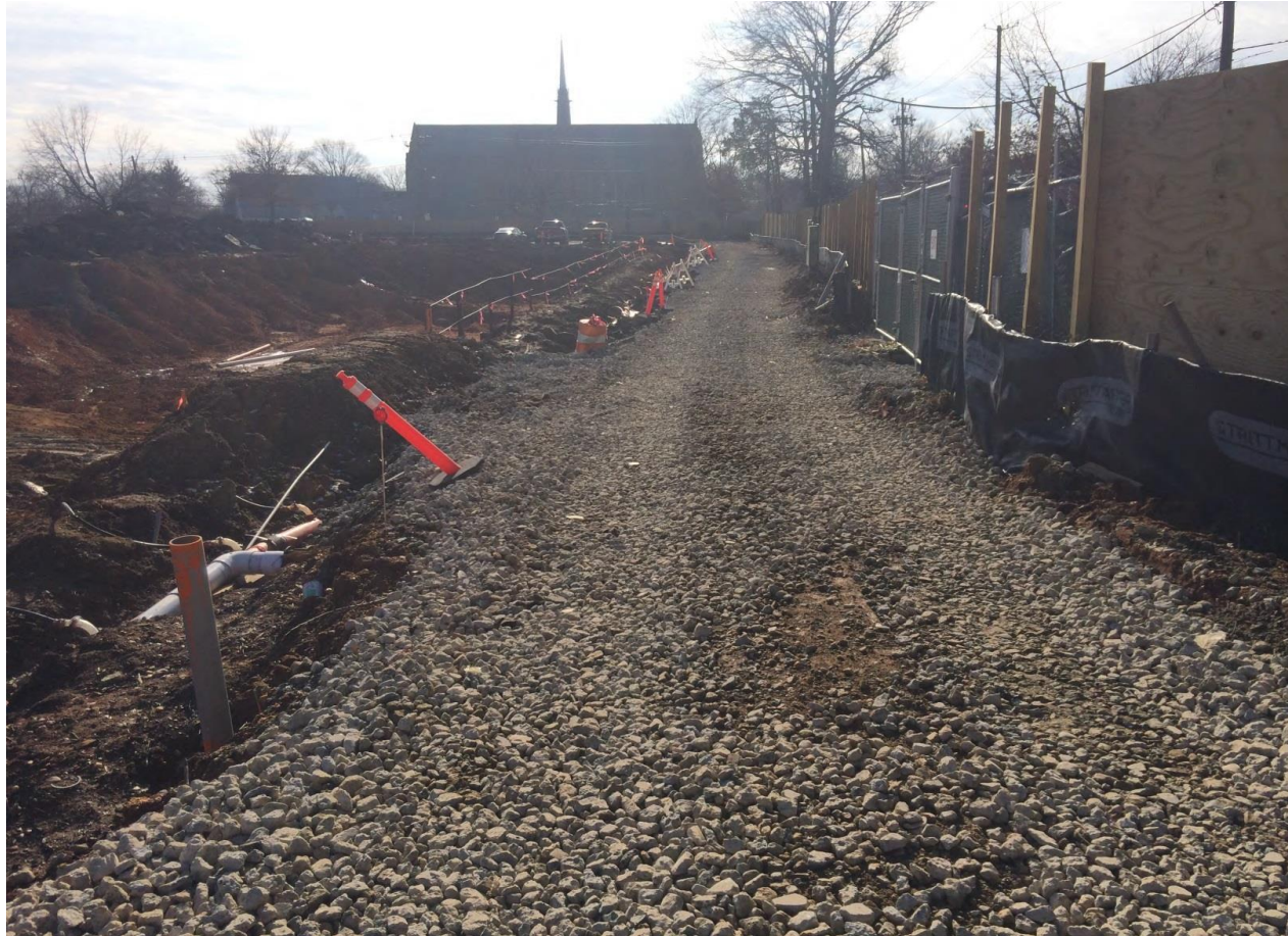
Excavation (facing south )
