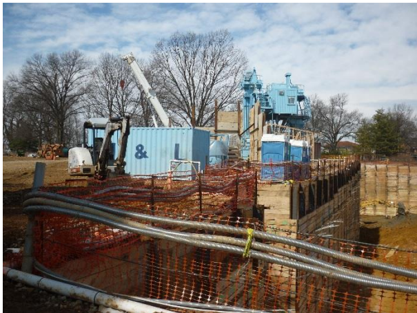
Concrete Batch Plant
