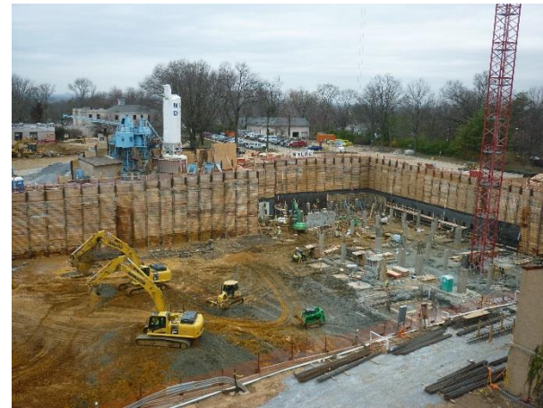
Garage Structure Construction
