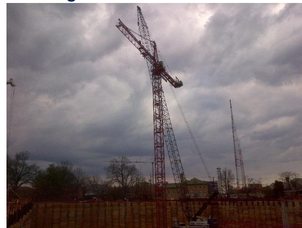
Tower Crane Installation
