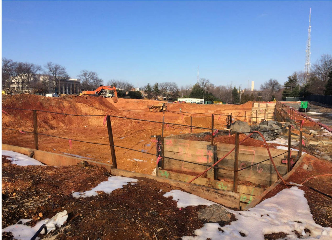
Excavation (facing north)
