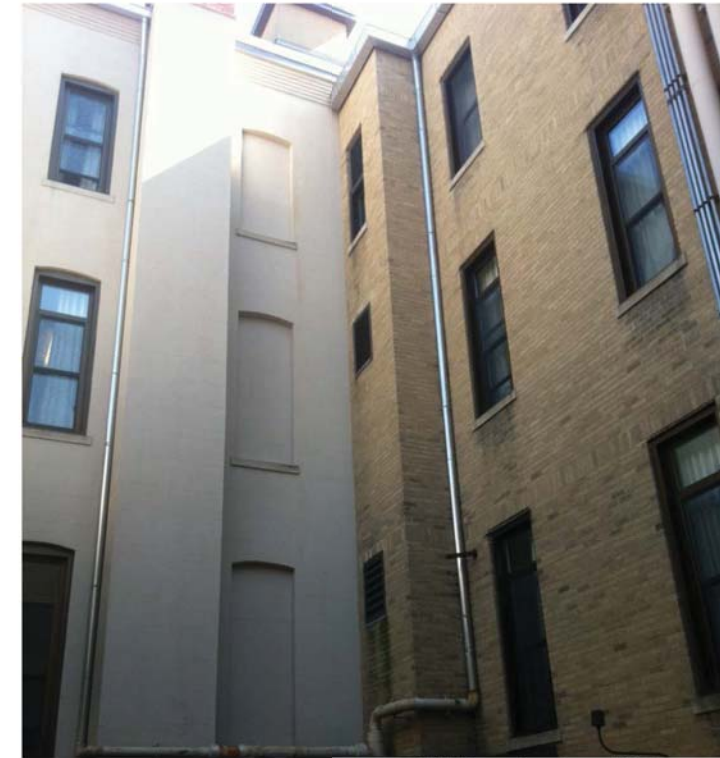
Existing elevator at SE corner
