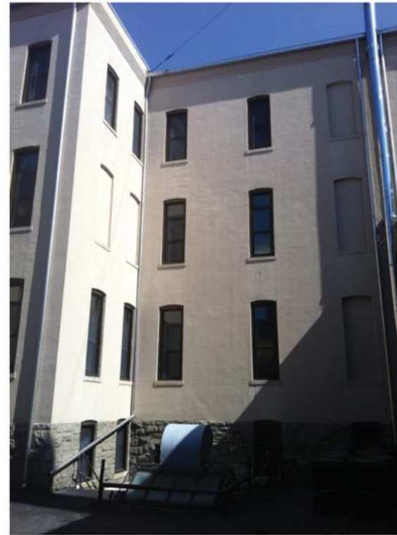
Existing conditions at NE corner
