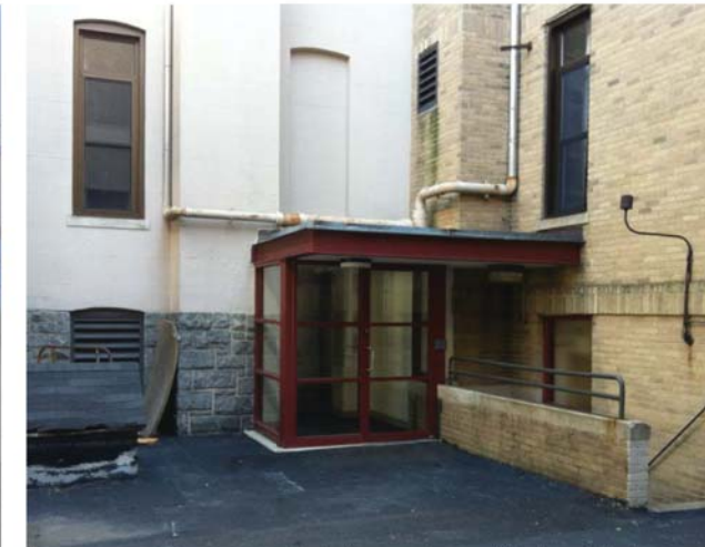
Existing entry vestibule at SE corner
