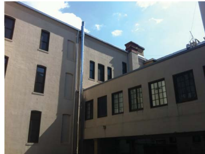
View of existing bridge connection
