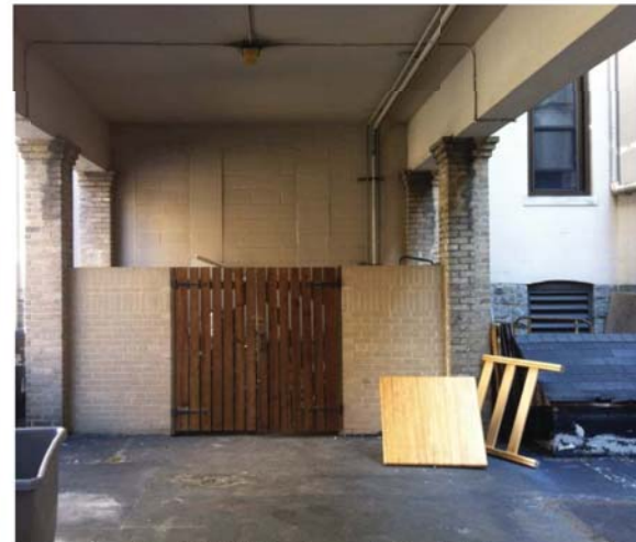
Capital Hall below existing bridge connection
