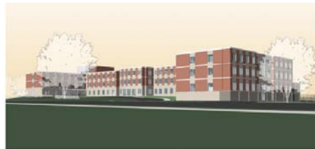
AMERICAN UNIVERSITY NEBRASKA HALL ADDITION NEBRASKA AVENUE FACING SOUTH 01.18.2011 LITTLE
