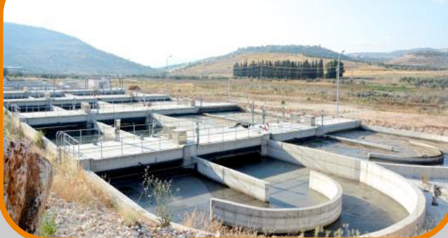
Nablus West Treatment Plant
