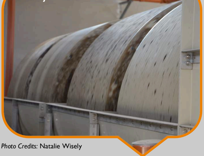
Al Taybeh and Ramoun Treatment Plant
