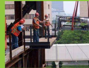
Workers guiding the MEP corridor racks onto the floor
