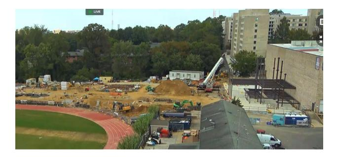
**Utility work** remains underway for the next 2 weeks completing the installation of the main water line for Meltzer as well as the building's main electrical conduit. This work temporarily limits access to the campus roadway adjacent to Leonard Hall. Fencing has been installed as a safety precaution and directional signage was placed along the fence to guide pedestrians through the area.
