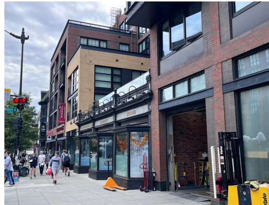
Retail and Building Entries
