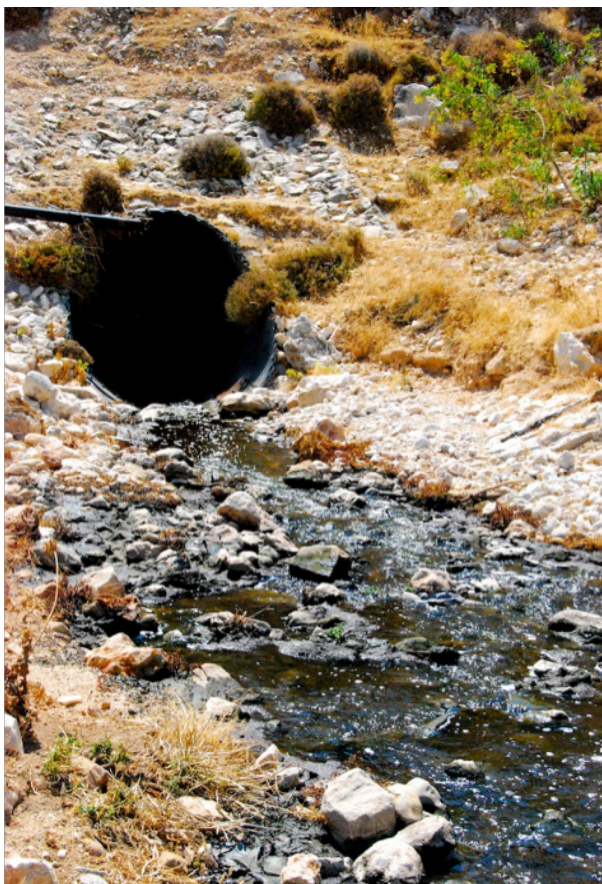
Sludge discharged from a Palestinian wastewater treatment plant (photo credit: Moses Jackson)
