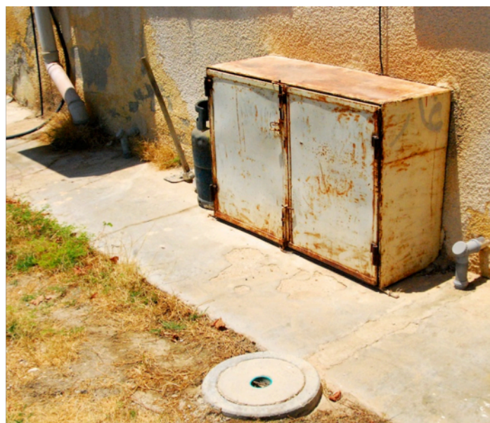
Piping is added to separate graywater from black water at the household level (photo credit: Moses Jackson)
