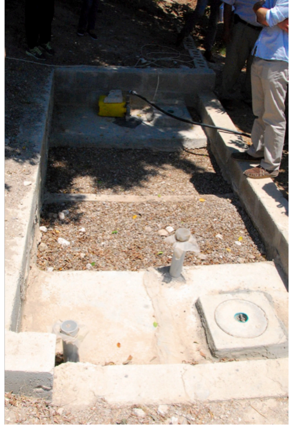
Graywater treatment system installed in Al 'Oja (photo credit: Moses Jackson)
