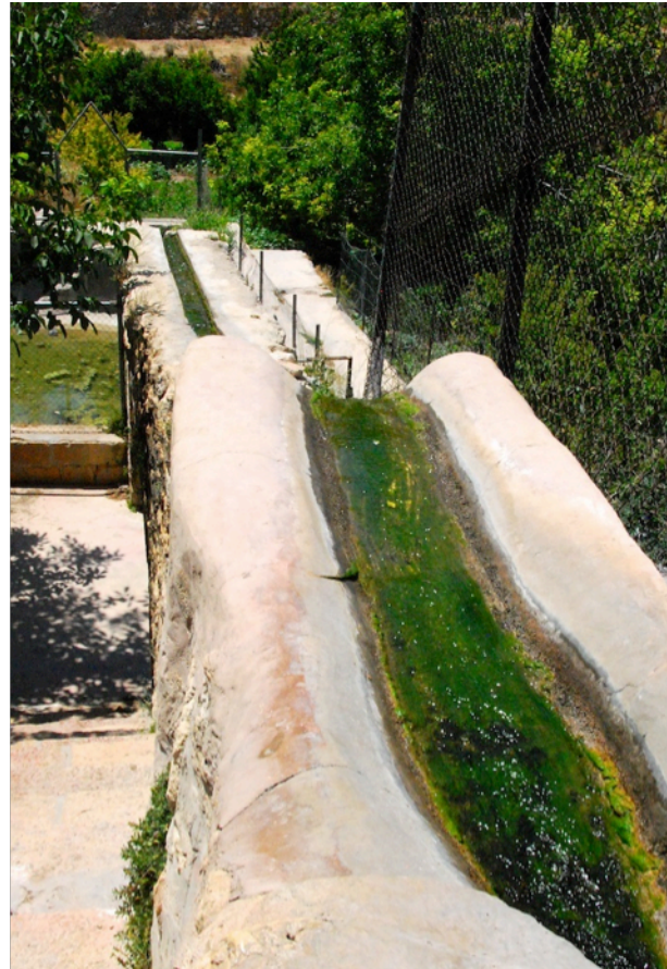
Roman-era water conveyance system in Battir (photo credit: Moses Jackson)
