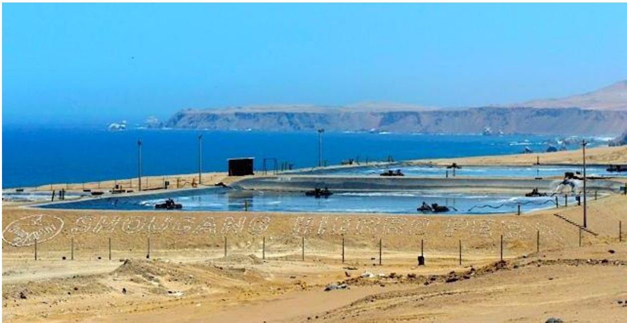
Oxidation ponds in Shougang's wastewater treatment facility located outside of Marcona Photo credit: Alison Minarcik
