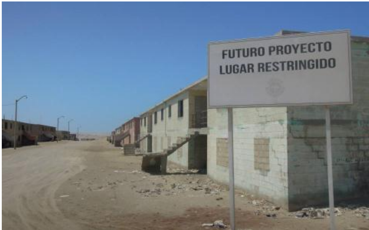
A faded sign stating “Future Project” and “Restricted Area” with Shougang’s company logo.
