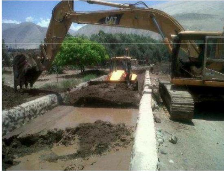
Road Construction in Caravelí Photo credit: Espinoza Colan and Serrano Guevara
