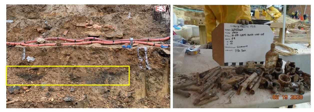
Photo of North Wall of PSB Foundation Excavation with yellow box showing Black AUES Debris layer about 1 foot below the former PSB basement slab elevation. During the PSB Foundation excavation, AUES Debris was observed extending beyond the excavation wall. Examples of AUES Debris recovered: broken glass, glass jars, test tubes, ceramics, and metal pieces. No Chemical Warfare Agent was detected.
